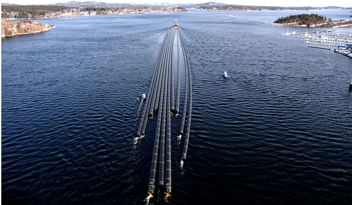
Departure of eleven OD1600 and OD2100 mm pipes, lengths between 500-600m.
