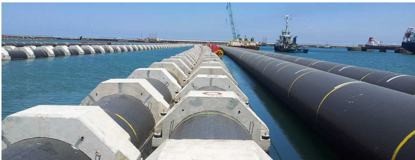
Typical pipe collar weighting for marine installation
