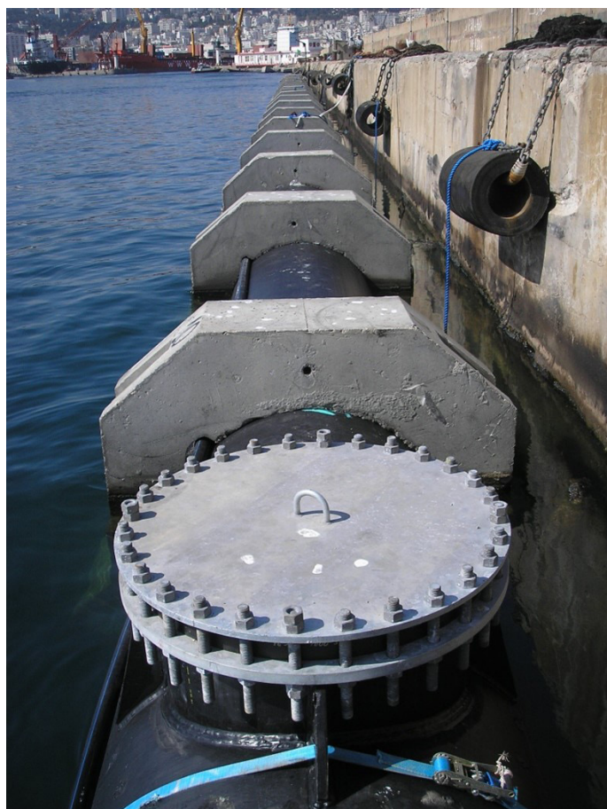
Completed saddle fitting with temporary blank flange
